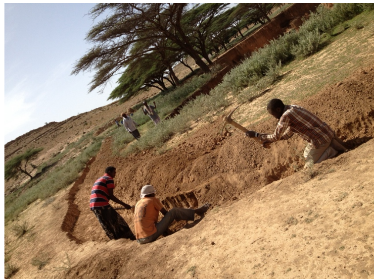
2. DURING THE WORK
